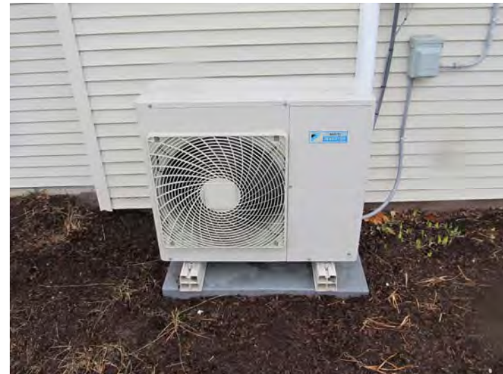
Exterior condenser for one of two recently installed heat pump systems serving interior common areas at community/office building
