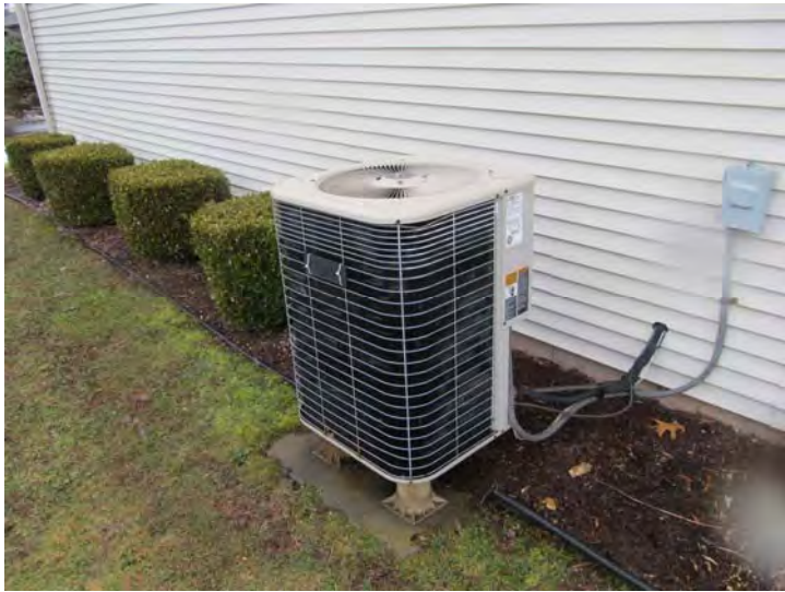
Exterior condenser serving cooling needs within management office suite
