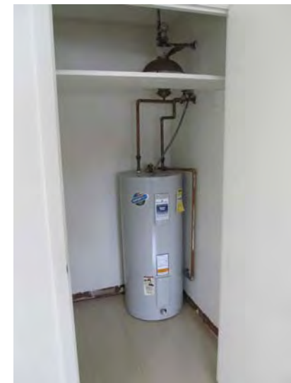
Typical unit-level electric domestic hot water tank
