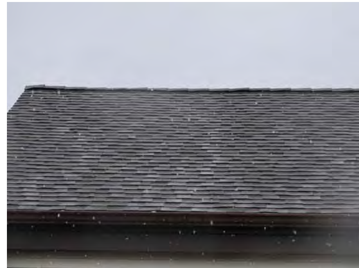
Typical architectural-style shingles found on roof surfaces at all buildings – No problems noted
