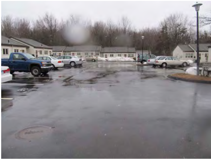
Asphalt paving at access drive and parking area is newer and in good condition
