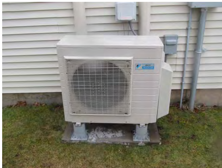
Typical exterior condenser for heat pump systems that were recently installed in all units
